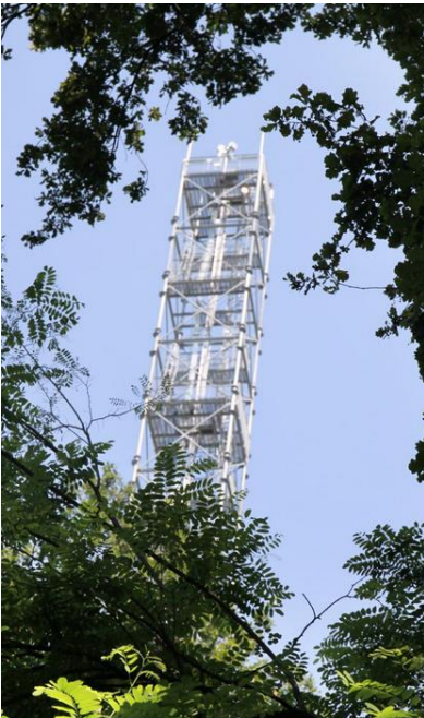
Atmospheric Observatory Tower at JRC Ispra site (Italy)
